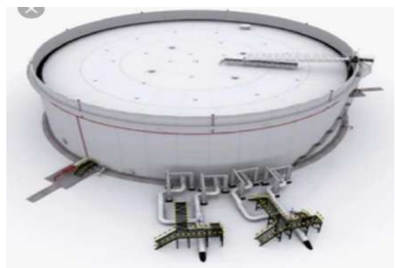
Figure 2: Floating roof tank
