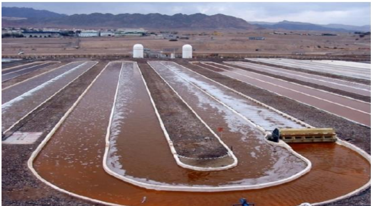
Figure 7: High rate algal pond in Arizona, USA. Sources: Renewable Fuel & Energy B.V. (62)
